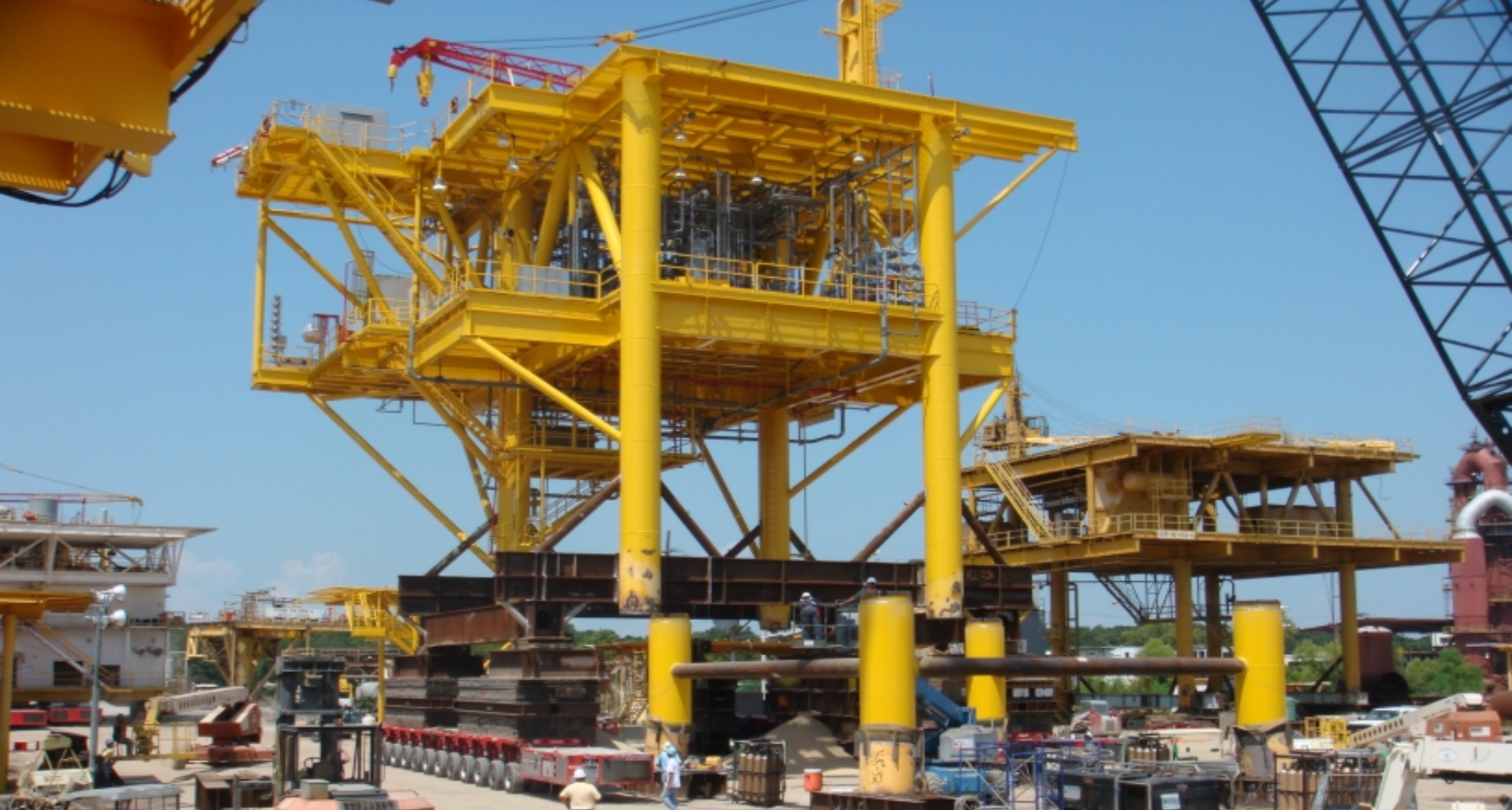
The deck begins its move forward to mate with its waiting new legs.
