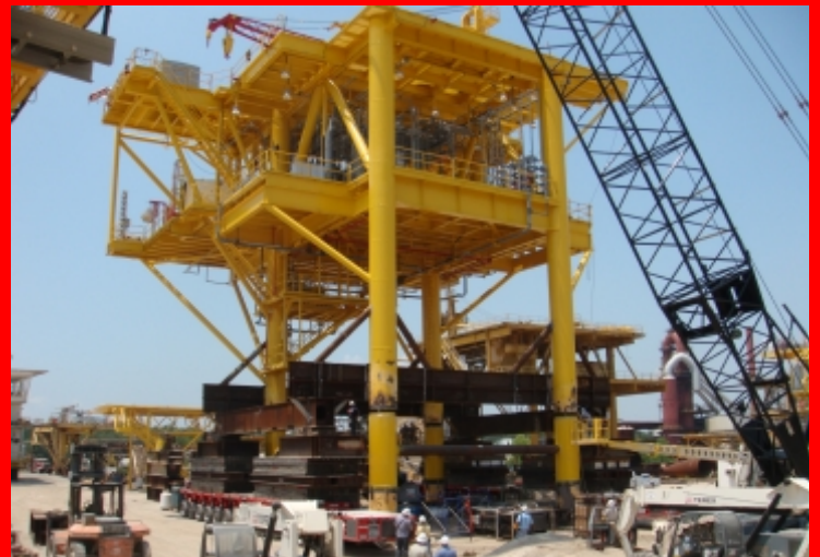
Ready to lower onto the new legs
